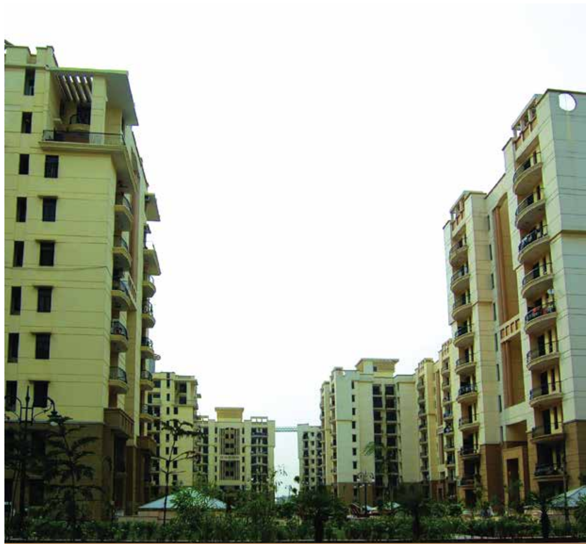
Actual picture shot on site of Purvanchal Silver City I
