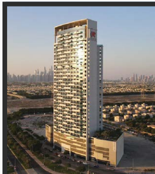
Al Jawahara Tower JVT, Dubai
