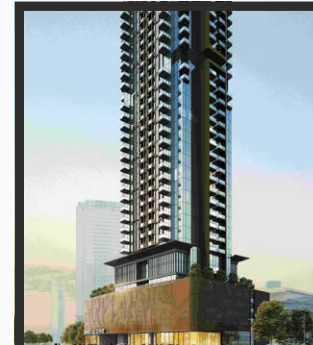
Seslia Tower JVT, Dubai
